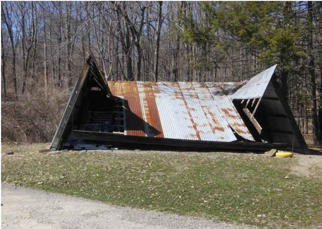
This is the hanger right opposite the ticket booth. The wind pickup up the roof and blew out the walls. It was not too bad but the heavy snow loads this winter brought the roof to the ground. This is on the Top of the list of things needing fixing at the Aerodrome as it houses at least 3 of their vehicles.
